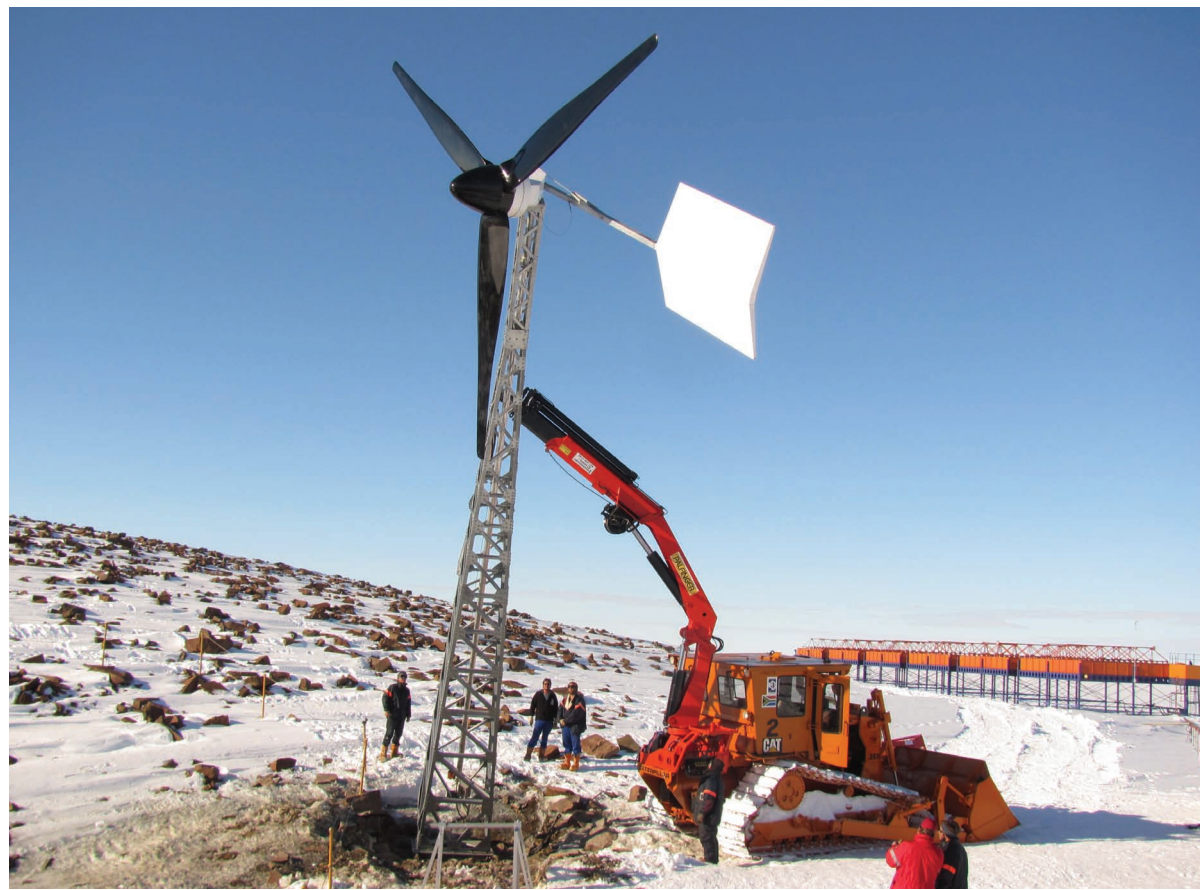
Members of SU's Faculty of Engineering erect the wind turbine that they designed at the SA base in Antarctica earlier this year. The lessons learnt on the icy continent can be applied in Africa, where extreme weather conditions also pose challenges.
